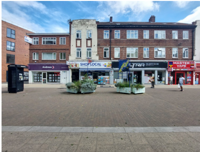
Degrading façade condition in North Street
