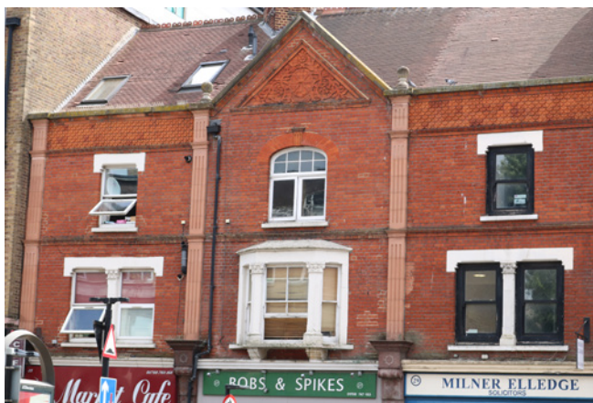
Visible rooflights to front roof pitches in the High Street
