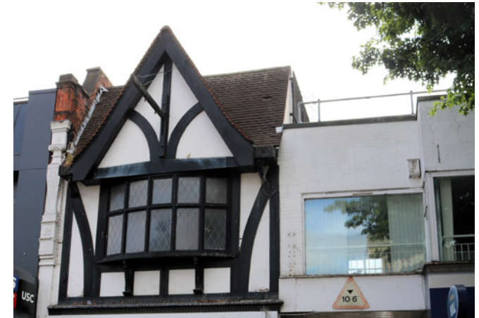
Cumulative impact of modern accretions to upper floors, Market Place
