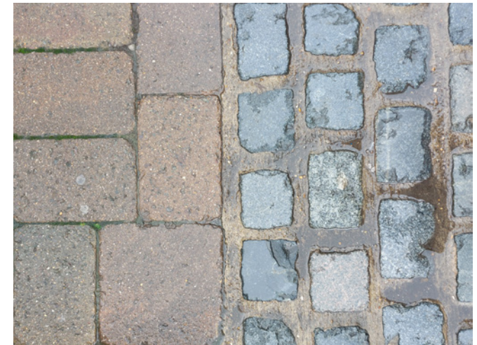
Surface detail on Market Place
