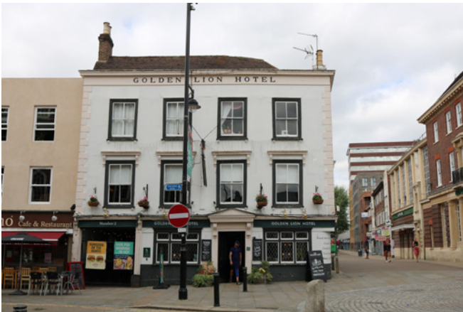
Georgian detailing to the southern façade of the Golden Lion pub, High Street.
