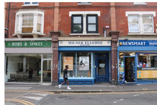
Original shopfront pilasters surviving in the High Street
