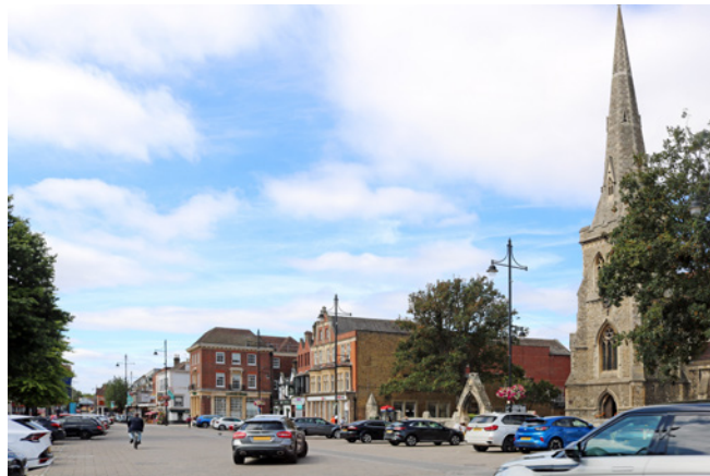
View looking northwest across Market Place, featuring St Edward's & historic commercial and public house frontages.
