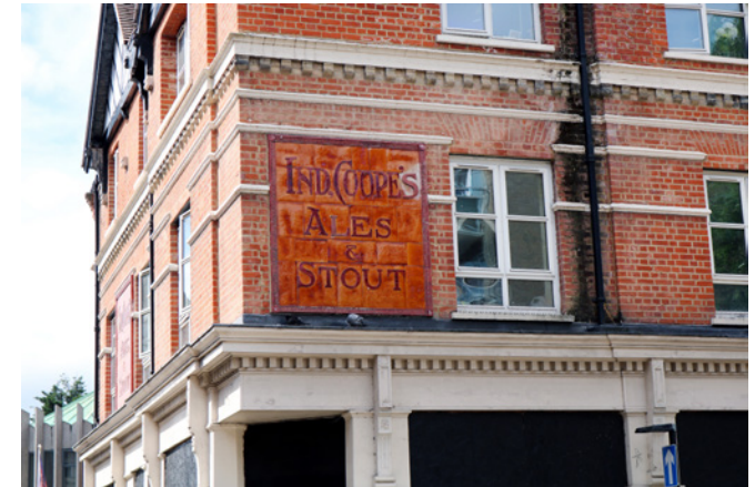
Detail of Woolpack decorative façade and signage, recording its origins as a Ind Coope public house.
