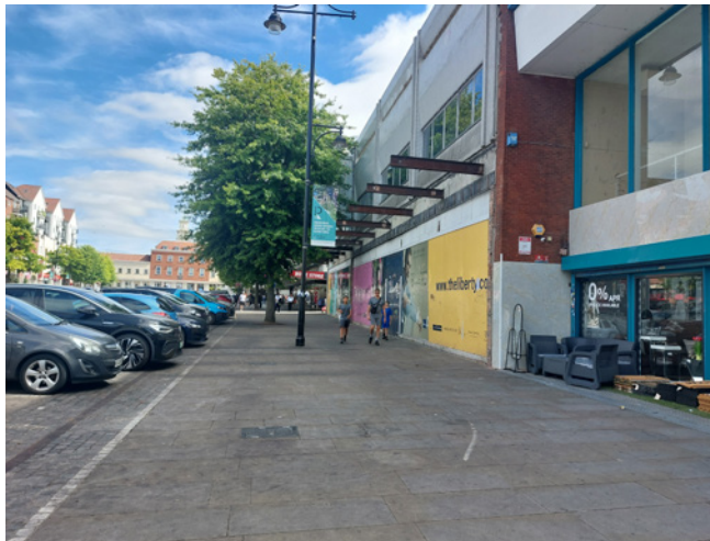
Vacant frontages in Market Place considerably detract from area character
