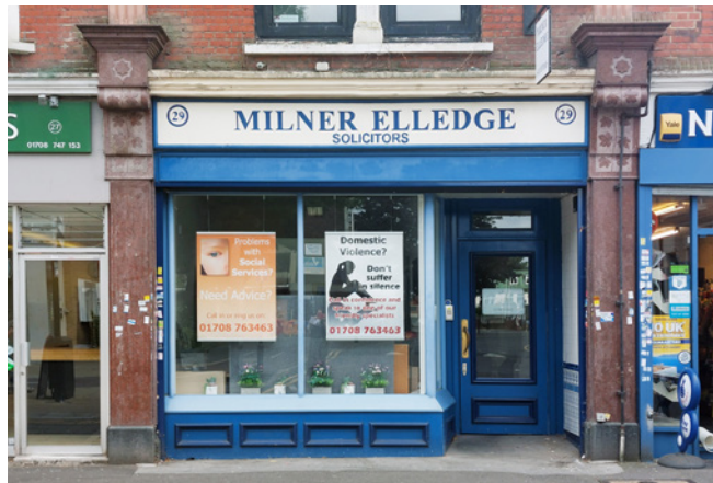
Shopfront at No.29 High Street.
