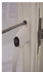
Figure 74 Tighten the top fixing using a Phillips screwdriver and push the cover cap back into place.
