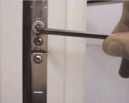
Figure 68 Allen key adjusted - rotate the roller using a 4mm Allen key.
