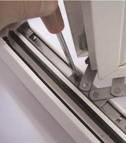
Figure 66 Adjustment screw.
