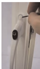
Figure 73 Carefully remove the top cover cap using a small flat-headed screwdriver.
