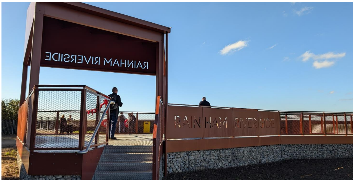
Figure 10. New Public Realm Improvement: Rainham Riverside
