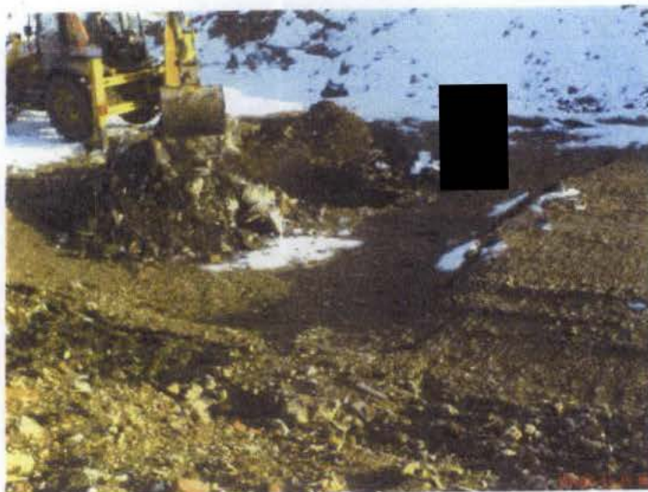
Plate 3: Area of Subsidence with Snow Melt Over Area of Recent Waste
