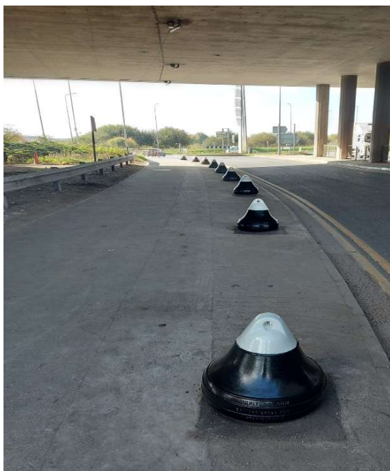
Figure 11. New bell bollard installation and planting
