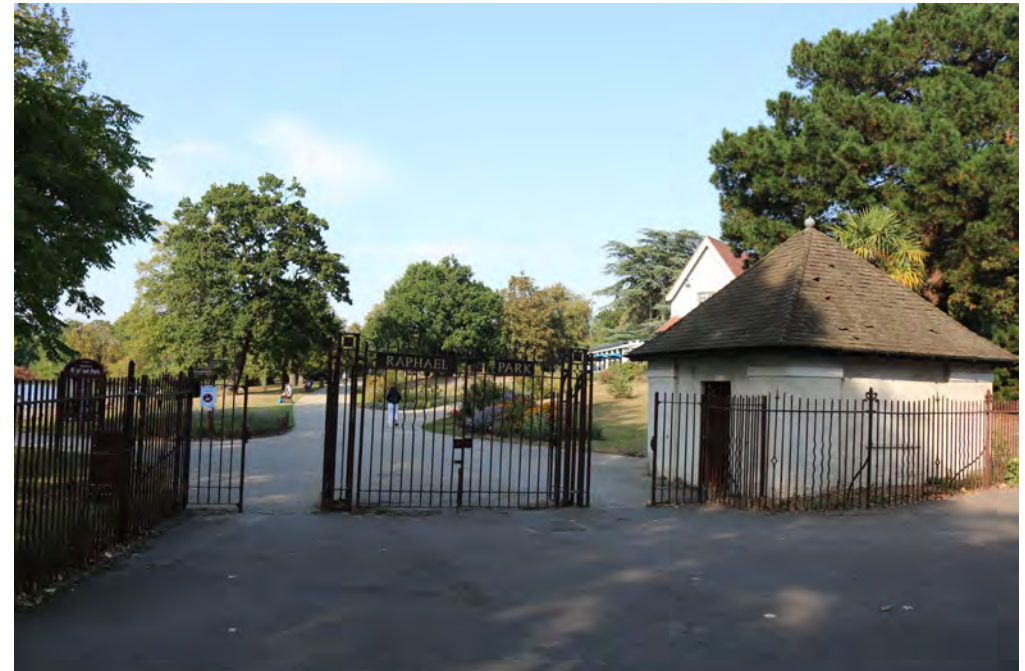
Raphael Park entrance gates and railings, Main Road
