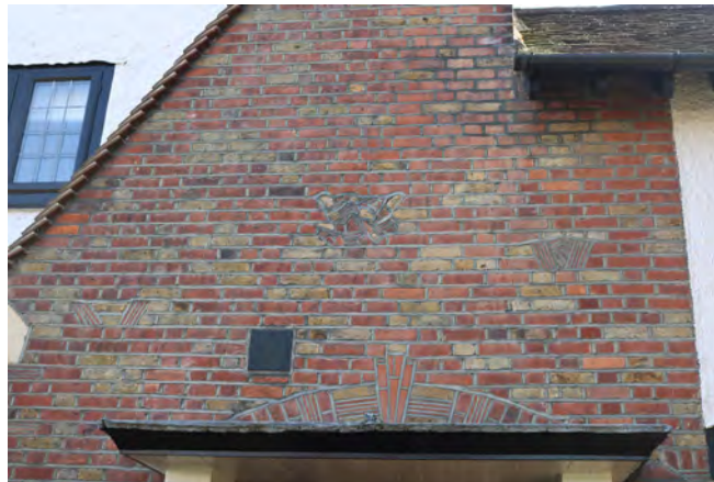
Detail of subtle decorative brickwork above main entrance at No.32 Reed Pond Walk
