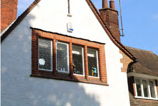
Horizontal window arrangement with brick mullions, Parkway
