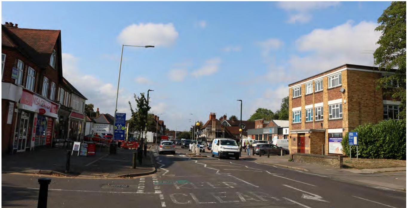
View from east end of Main Road, looking west into the conservation area.
