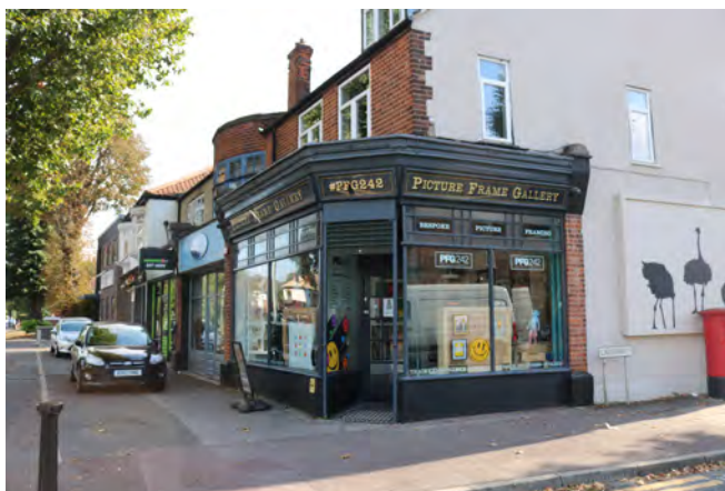
Shopfront with historic character at corner of Main Road & Crossways
