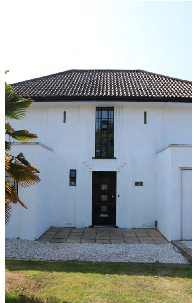
1930s front elevation detailing, Heath Drive
