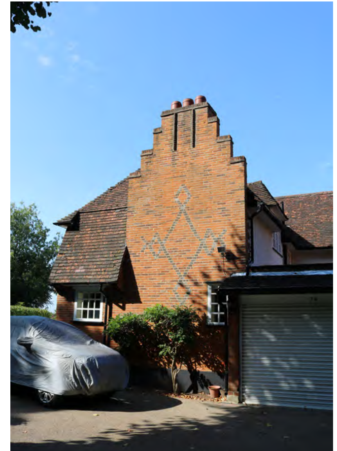
Detail of polychromatic brickwork set within the chimney breast at No.74 Parkway
