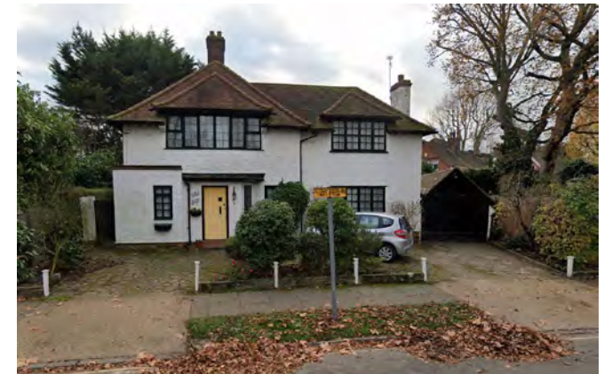
Mismatched window replacement, Balgores Crescent
