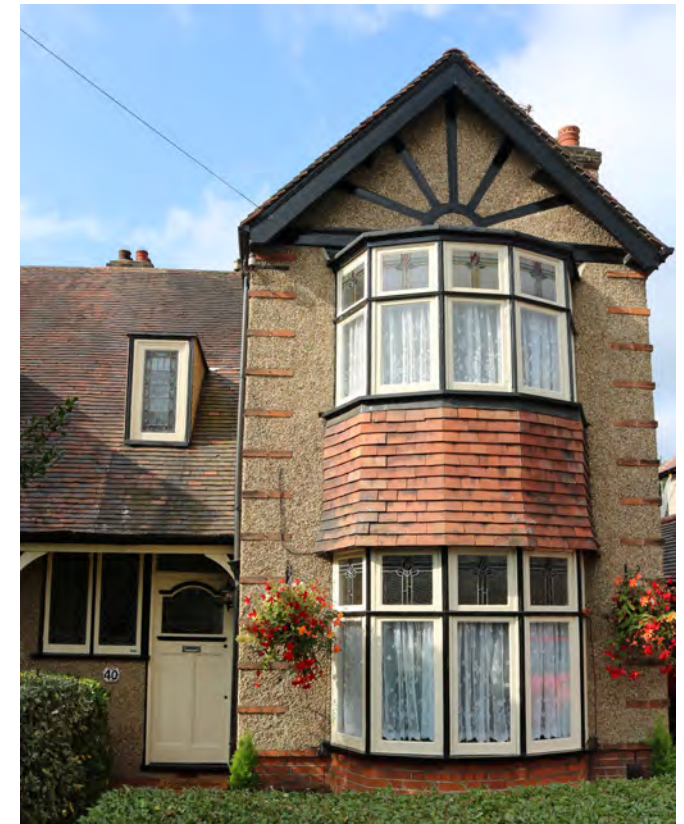
Intact timber window arrangement, Crossways
