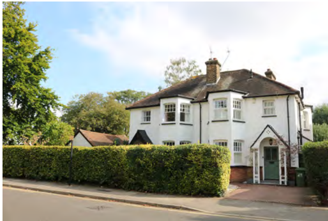
Semi-detached houses on Crossways
