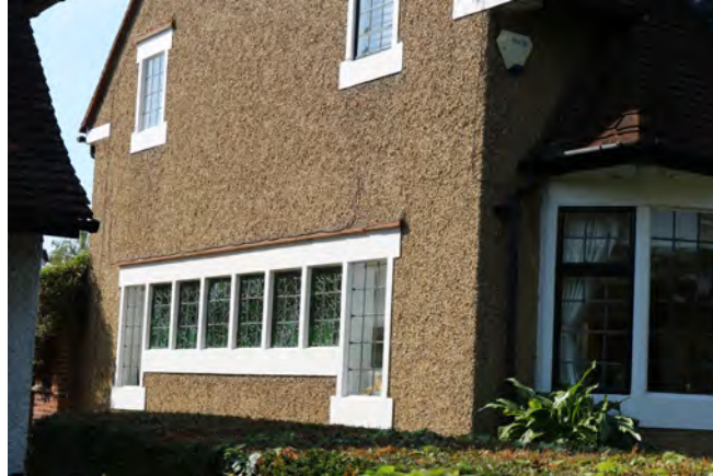
Decorative window to return elevation, Heath Drive
