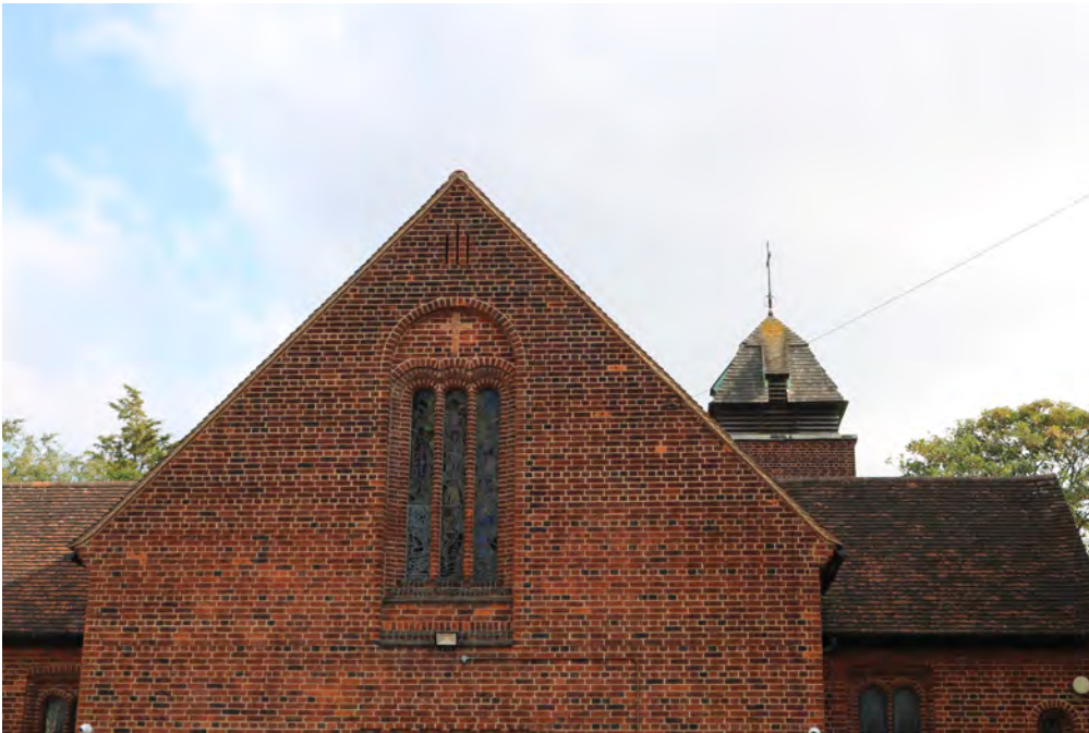
Detail of brickwork at St Michael and All Angels church
