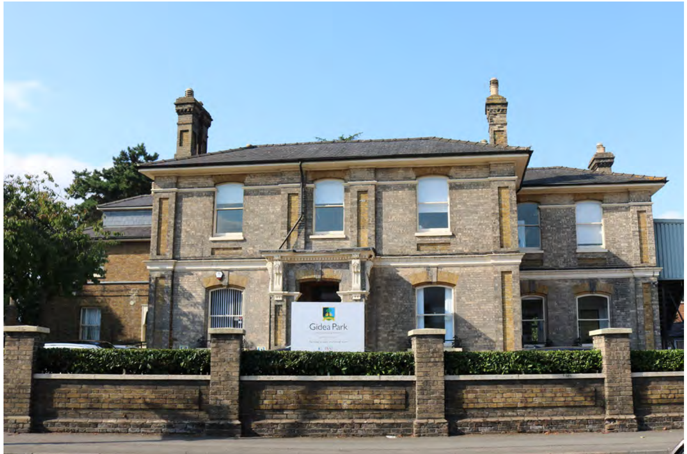
Balgores Lane façade of the Gidea Park Preparatory School.
