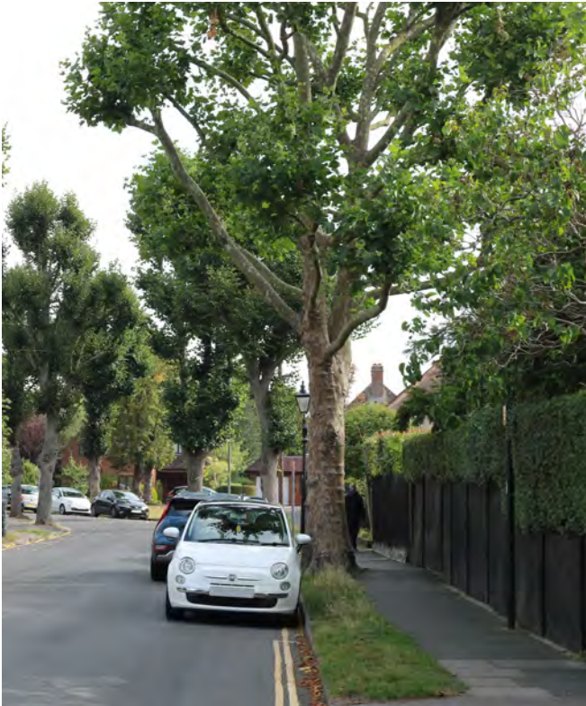
Street and pavement surfacing on Balgores Crescent.
