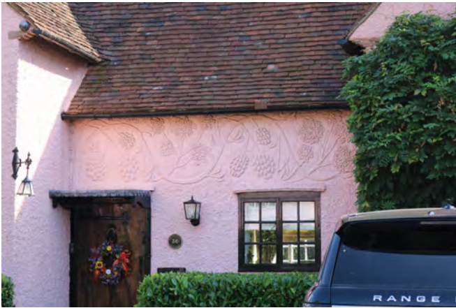
Detail of front elevation plasterwork.
