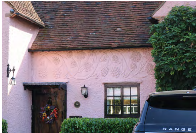
Detail of decorative plasterwork to No.36 Reed Pond Walk
