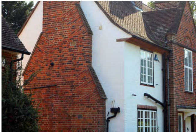
Detail of chimney brickwork.
