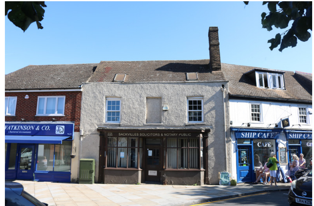
Visible rooflights at the village centre
