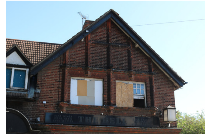
Detail of upper storey of the Bell Public House.
