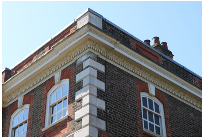
Detail of decorative stonework deployed at Rainham Hall, Grade II*
