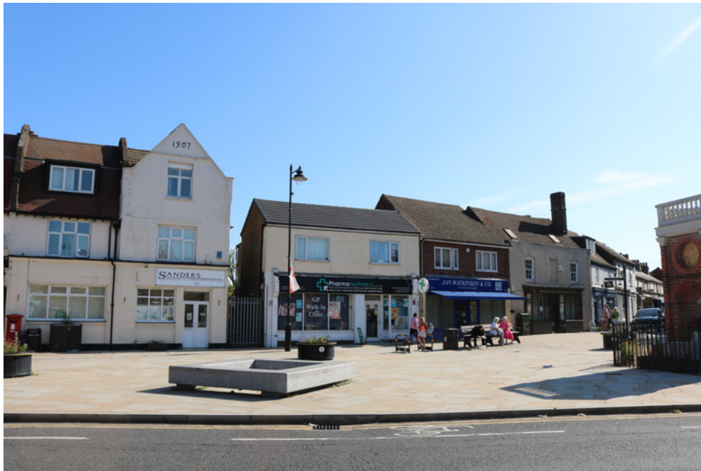
Low-quality window replacement is evident across prominent conservation area façades
