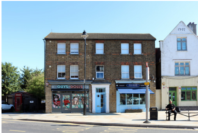
Shopfronts within No.24-28 Bridge Road, built c.1897
