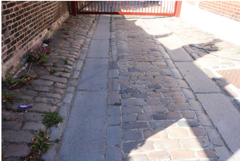
Detail of historic setts on off-street entrance to Redbury House.
