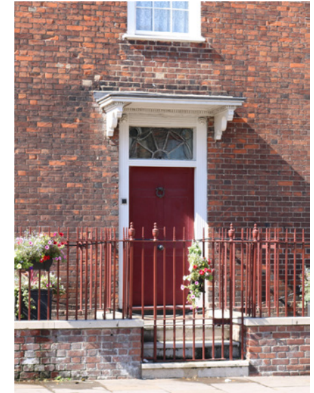
Detail of entrance canopy at Redbury.
