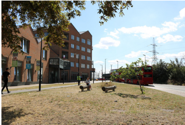
View of public realm between the library, bus depot and railway.
