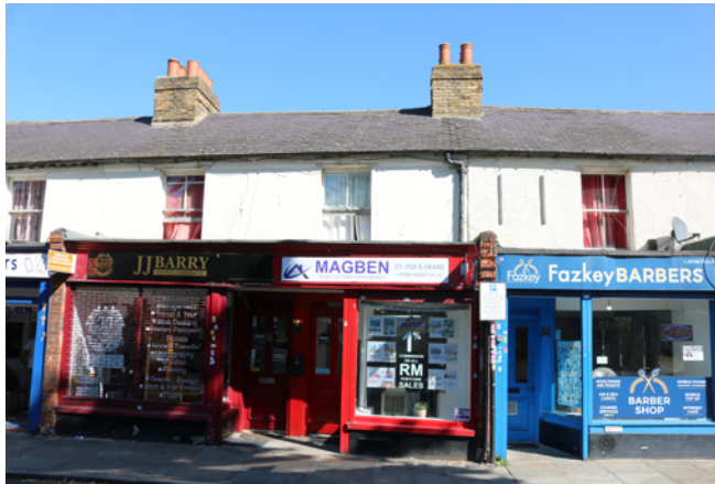
View of shopfronts at No.19-23 Upminster Road South, showing late 19th century extensions to early 19th century terraced cottages.
