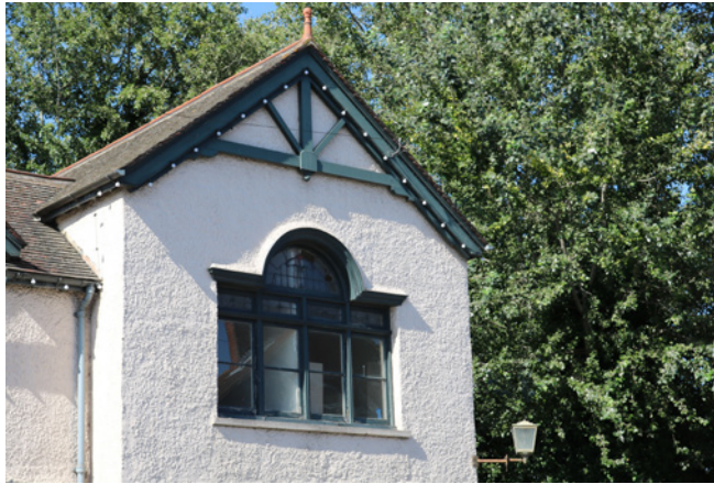
Detail of first floor window of the Angel Public House.
