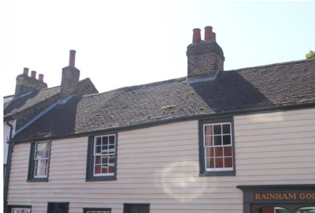
Detail of traditional weatherboard and roofline of No.2-8 Upminster Road South, Grade II.
