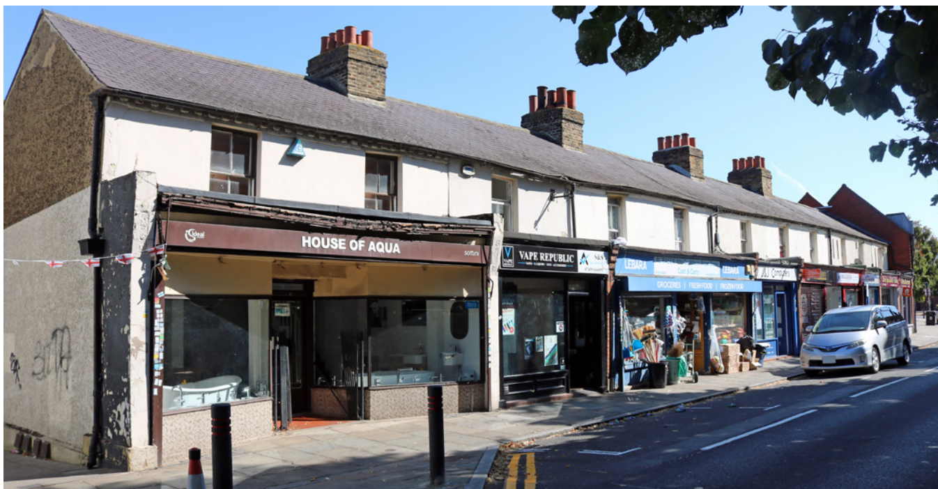
Overlarge glazing without subdivision is generally inappropriate for a shopfront within a historic frontage
